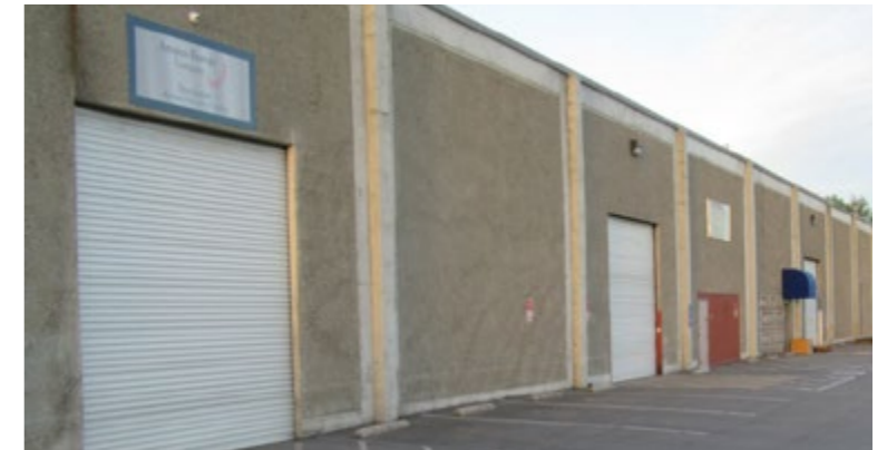
Pump Remanufacturing Center – Stockton, California
