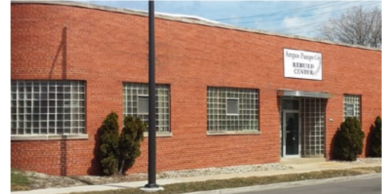
Pump Remanufacturing Center – Milwaukee, Wisconsin
