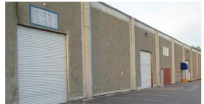
Pump Remanufacturing Center – Stockton, California
