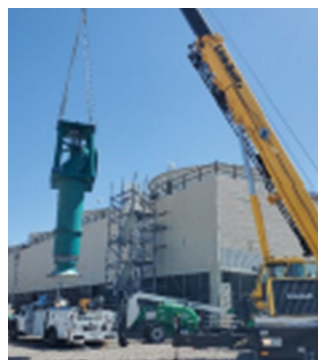
Circ Water Pump Replacement
