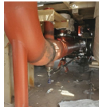
Main Steam Header Replacement
