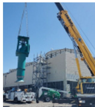
Circ Water Pump Replacement
